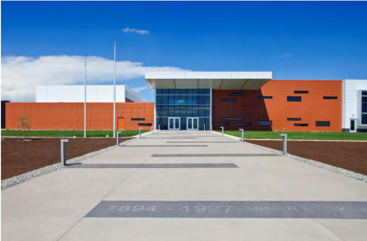
Completed Northern Colorado Springs Readiness Center. Sheet metal panels on soffit, terracotta panels and insulated panels on the fascia.
