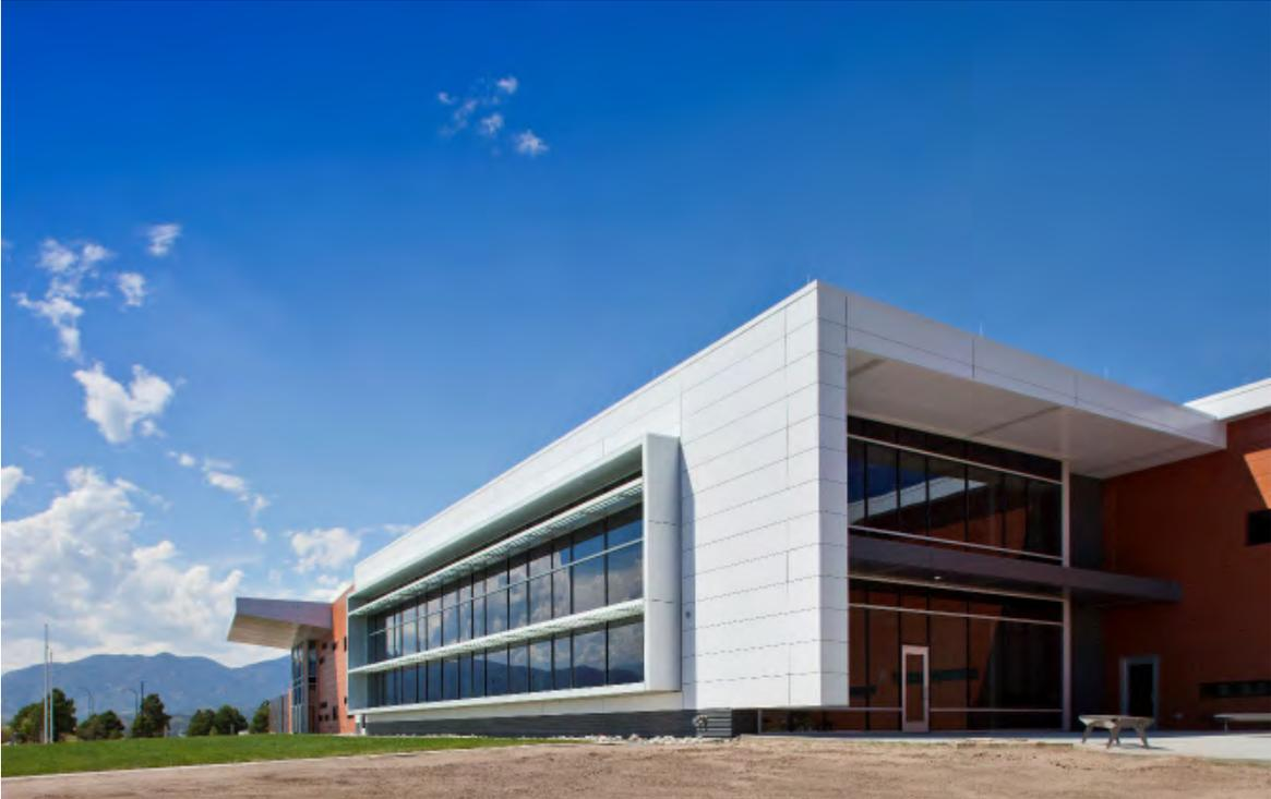
Architectural insulated panels. On right side, soffit panels that are sheet metal panels.
