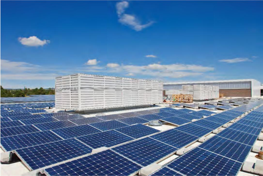
Photovoltaic solar panels installed on membrane roofing.
