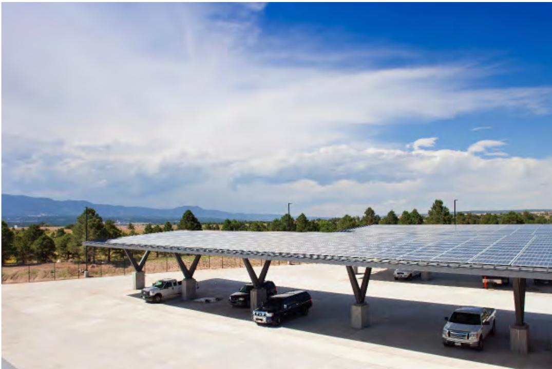
Carports are covered with photovoltaic panels. Seam metal roofing is underneath the panels. Sheet metal soffit and fascia panel installation.
