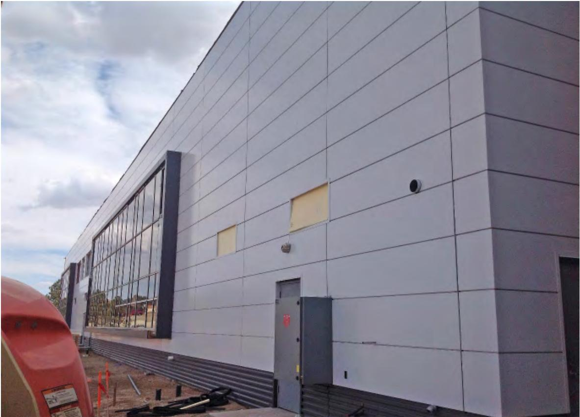
Architectural insulated panel's custom sized showing two different panels.
